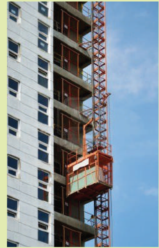
Lift to take materials
